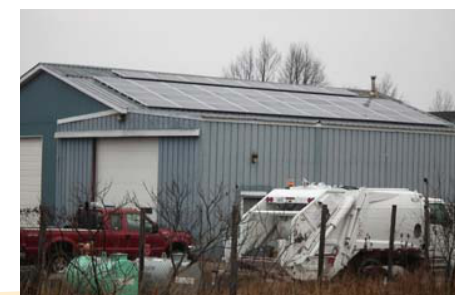
SOLAR PV INSTALLED ON A PUBLIC WORKS GARAGE
